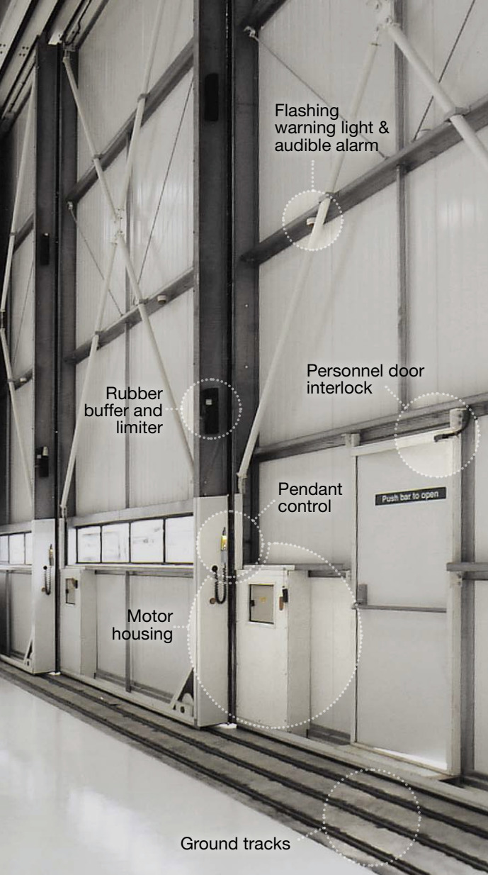
Interior view of one of our door systems, consisting of four independently driven door leaves; three are glazed.
