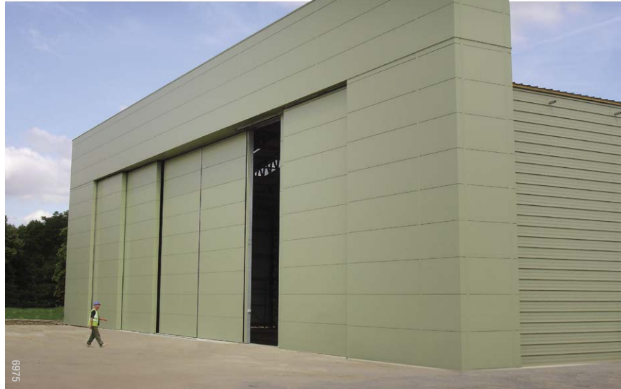
Hangars doors clad in horizontally laid microrib composite panels to give a clean appearance on the inside.
