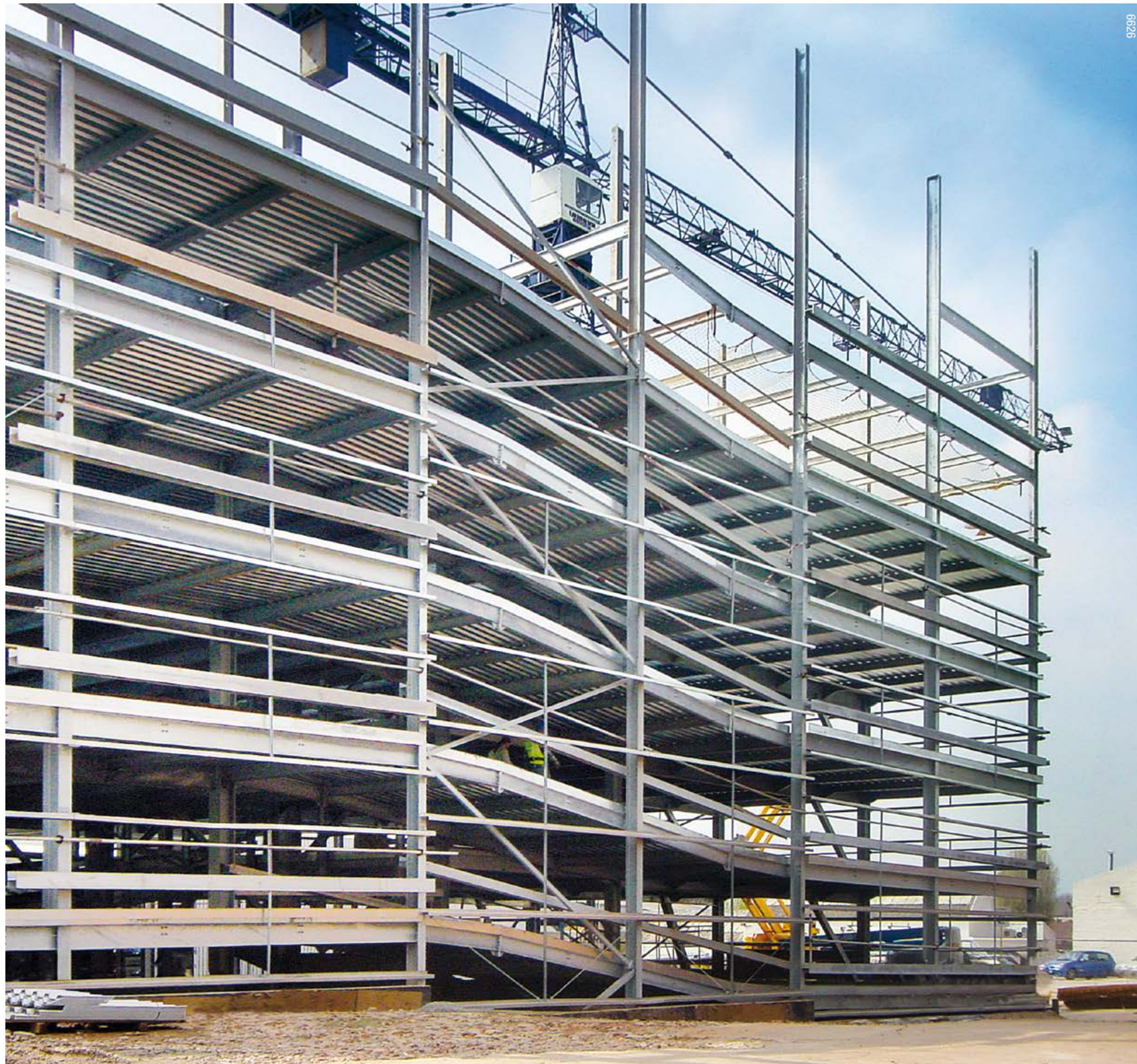
BMW Car Park, Coventry, UK The steel frame design produces clear open floor spaces.
