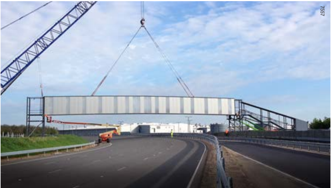
Above: Pedestrian bridge under construction. Above right: The crossing via our highway bridges is via a pedestrian walkway which is kept separate from the main highway section
